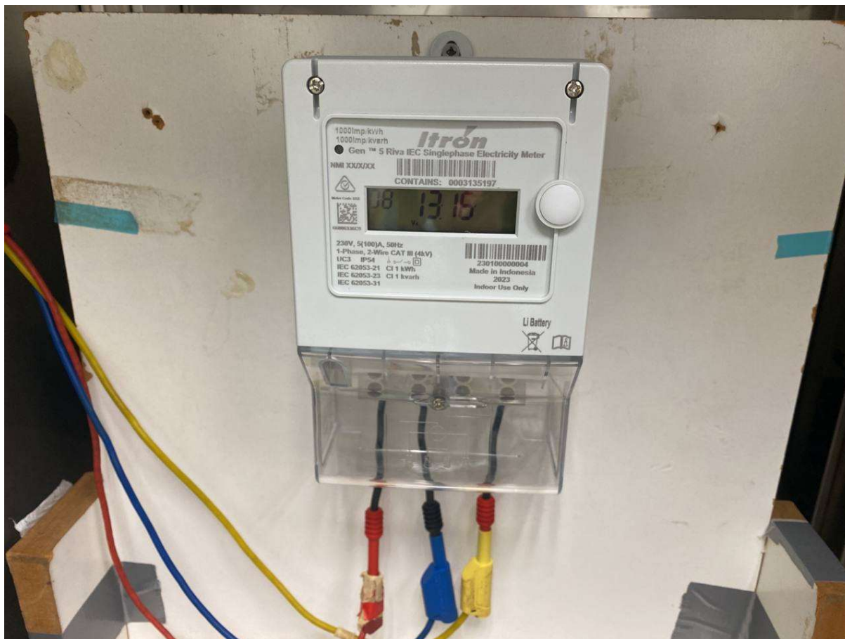
Figure 3: Test of Crystal-Controlled Time Switches with Temperature Setup
